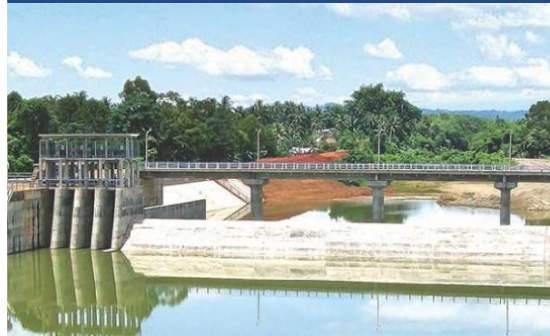
Public access to basic service infrastructure
